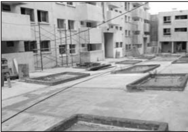
COVIREUS cooperative, currently under construction. Picture courtesy of Mariana Oliver.
